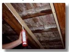
7. Fill the joints between batten and rafters with GUTEX caulking along the entire length of the joints.
