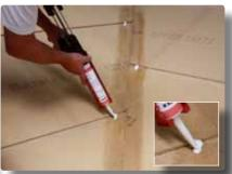
5. Fill the joint with a sufficiently large bead of GUTEX caulking.
