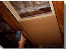
8. Fasten the GUTEX Multiplex-top boards to the batten.
