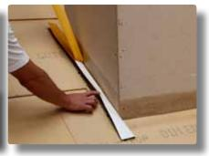
3. Apply GUTEX adhesive tape without air blisters or wrinkles over the joint, pressing on the caulking to smooth and flatten it.
