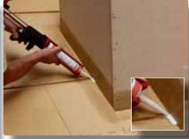
2. Fill the joint with sufficient caulking material.
